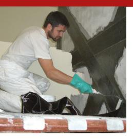
TECHNOKOMPOSIT is the acronym to define systems specially designed to perform structural and other reinforcements of buildings, subject to serious degradation, also due to earthquakes, through the use of the technology of composite systems (reinforced fibre - FRCM) based on carbon fibres, basalt, glass and aramid.
