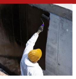
SYNTECH TARPOX is a two-component solvent-free epoxy-hydrocarbon resin based product. SYNTECH TARPOX has excellent characteristics of waterproofing, elasticity and flexibility. SYNTECH TARPOX is among the products most used for waterproofing and cold protective treatments of concrete and steel products.
