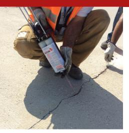
Syntech Roadware is a high penetration two-component hybrid urethane which, combined with quartz, produces a hard and instant polymer to repair cracks and crevices in concrete floors.
