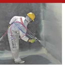
Syntech Poliurea Spray - FC is a pure aromatic polyurea specifically designed for contact with food substances and drinking water. 100% solid does not contain VOC and can only be applied by spraying using suitable bimixer machines. It is aromatic and is characterized by a high degree of elongation. It is a coating elastomer obtained from the reaction of an aromatic type isocyanate with an amine. PURE POLYUREA SUITABLE FOR FOOD CONTACT
