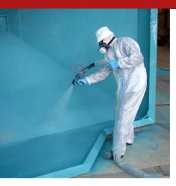
Syntech Poliurea Primer – Epoxy Metal is a two-component primer based on epoxy resins free from solvents, used to promote adhesion, as a surface sealant for concrete, applied as a substrate for works with polyureas on metal surfaces and epoxy and polyurethane coatings.
