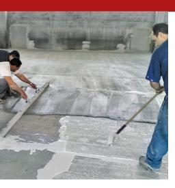
A two-component epoxy system based on epoxy resins in aqueous dispersion and solventfree. It is ideal for completing protective, transparent treatments with a consolidating action and anti-dust effect on industrial concrete flooring, with good mechanical and chemical resistance, especially in reference to contact with oils and solvents. This product also serves well as a primer for casting joints between old and new concrete flooring.
