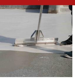
A three-component formulation, with a fluid epoxy resin base in aqueous emulsion (A + B) to be mixed with the third component (C) consisting of white cement and micro-quartz, specially designed to be used as a primer for cementitious surfaces in the presence of humidity and in conditions of hydraulic counter-thrust. Generally referred to as "wet-bonding", it is particularly suitable as an anti-humidity barrier for the subsequent laying of parquet.
