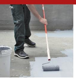
Colored two-component finish, permeable to water vapour, based on epoxy resins in water dispersion. Ideal for the pigmented coating of industrial floors and concrete constructions in general with residual humidity and without vapor barrier. Surfaces treated with Syntech Pavicrom SBV are easy to clean and guarantee excellent resistance to mechanical wear, as well as being highly resistant to water, alkaline solutions, detergents and hydrocarbons (petroleum, diesel, petrol, etc.) .
