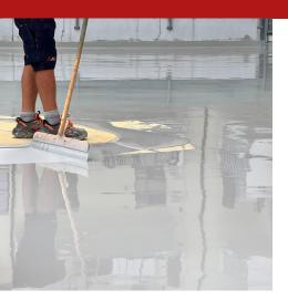
Two-component coating based on epoxy and polyurethane resins; for the coating, waterproofing and elastic protection of roofs, terraces, pavements, stairs, car parks and surfaces that are cracked or subject to micro-cracks and crazing.
