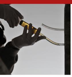
A two-component pure epoxy adhesive that is fluid with a low viscosity, free from fillers and solvents, being specific for high performance structural consolidation injections in crumbling masonry, degraded concrete, aging screeds and industrial flooring, cracked plasters and mortars and so on. It is ideal for securing bars, clamps and tie-rods. It is also perfect for the deep consolidation of wooden materials and other types of porous materials, with impregnation by brush or roller.
