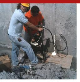
Manual single-piston pump, self priming, simple effect, to inject polyurethane and epoxy fluid resins. The maximum pressure that can be delivered by the pump is 40 bar. The flow rate is 1 litre in 55 cycles.
