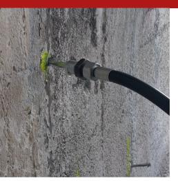
Connection element between the flat head injectors and the pumping tube of manual or electric pumps, used to block water infiltration by injections of water-reactive polyurethane resins.
