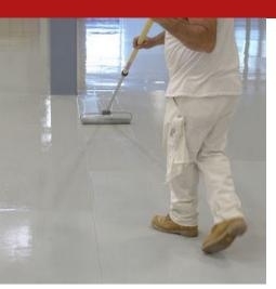
Syntech Flexipur is a two-component aliphatic elastic polyurethane resin in the solvent phase, with excellent characteristics of chemical resistance and flexibility, ideal for the protective finish of both new and restored reinforced concrete structures. Syntech Flexipur is applied by roller or spray (airless) creating a film-forming coating with high protective capacity and resistance to cracking (crack bridging ability).
