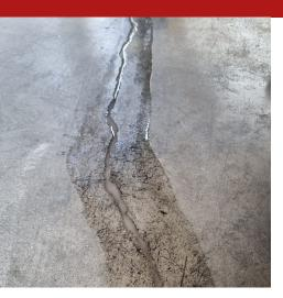
Two-component, high-solid, epoxy resin-based filler that can be used with quartz and/or inert fillers to repair cracks in concrete floors.
