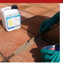
A two-component, fine cementitious grout with a fluid plastic consistency for grouting uncovered joints or filling and finishing static cracks, micro- and macro-cavities and so on between flooring tiles, before applying Protech Balcony for breathable non-film waterproofing operations on terraces and balconies.
