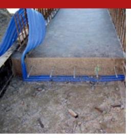
The Sealpvc SF 250 Bulb waterstop is a waterproofing PVC profile that is not hydro-expansive, having a thickness of 25 centimetres and equipped with a central and highly elastic bulb. It is used in dynamic joints for horizontal casting (slabs), in concrete structures, resting on the substrate beneath the reinforcement, in a position central to the casting.
