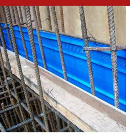
The SEALPVC SF 250 waterstop is a waterproof profile in PVC that is not hydro-expansive, having a thickness of 24 centimetres and high elasticity. It is used in static joints for horizontal casting (slabs), in concrete structures, resting on the substrate beneath the reinforcement.
