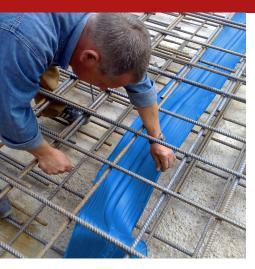
The Sealpvc RG 250 Bulb waterstop is a waterproofing PVC profile that is not hydro-expansive, having a thickness of 25 cm with a central and highly elastic bulb. It is used in dynamic joints for horizontal (slabs) or vertical (elevation walls) constructions, in concrete structures, in the central position of the cast.
