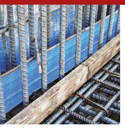
The Sealpvc RG 250 waterstop is a waterproofing PVC profile that is not hydro-expansive, having a thickness of 25 cm and high elasticity. It is used in static joints for horizontal (slabs) or vertical (elevation walls) constructions, in concrete structures, in the central position of the cast.
