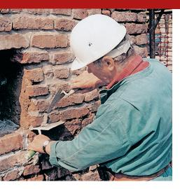
Adhesive high breathability and moldability mortar, based on hydraulic lime, for filling the vanishing points between elements in stone, brick, mouldings, decorative articles etc., in ecological building interventions, new buildings and in the restoration of vintage buildings and monuments. It can be added with earth colours, ornamental aggregates etc.
