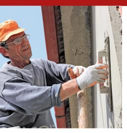
This macroporous, breathable, dehumidifying, fibre-reinforced plaster, with a base of natural hydraulic lime NHL 3.5, is for the dehumidification and hygrometric restoration of buildings and masonry, in works on green buildings, for new constructions and in the restoration of historic and monumental buildings.
