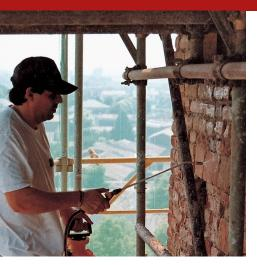
Reactive solution of mineral silicates, capable of forming binding and stabilizing compounds for hardening and consolidating treatments by reaction with hydrated calcium salts and moisture present in masonry, plaster, stone and concrete. Indicated in the preliminary treatments to the subsequent plastering or smoothing operations, of plasters and powdery mortars and wall casings in general, in green building interventions and in the restoration of period and monumental buildings.
