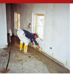
Walkable screed based on hydraulic lime, silico-calcareous aggregates with a maximum grain size of 5 mm and light aggregates with pozzolanic activity, fiber-reinforced with polypropylene and glass microfibres, used for the construction, with the addition of water, of resistant screeds and substrates , in green building interventions and in the restoration of period and monumental buildings.
