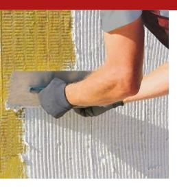
Single-component adhesive-skim coat based on hydraulic lime, special flexible polymers, rheological additives, water retainers, microsilicates with pozzolanic activity, spherical aggregates with low specific weight. To be used for leveling skims on various substrates, light gluing and as skim coat/adhesive for our special SANATEX membrane (on thermal bridges, damp and/or damaged masonry).
