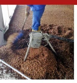
Binding, vitrifying, thick, syrupy solution of natural simple molecule minerals, for the production of insulating conglomerates, based on natural powdered cork, for ecological building interventions and in the restoration of vintage buildings and monuments.
