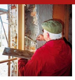
Adhesive, thixotropic, reinforced fibre compound, based on hydraulic lime, reinforced fibre, fast-curing, for fastening and anchorage, of wall bodies, structures, inserts, plates, frames, bars, sanitary, etc., in ecological building interventions, new buildings and in the restoration of vintage buildings and monuments.
