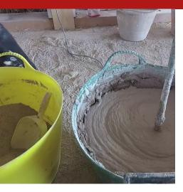
Sanafast is a specially formulated premix that, added during the mixing phase to our mortars (REPAR, GROUT, FLOOR, RINFOR lines) and to our natural hydraulic lime-based injection products (Sanafluens, Mikrosana), allows to accelerate the setting and hardening, with a much faster development of mechanical strength.
