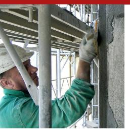
Thixotropic, anti-shrinkage, fibre-reinforced repair mortar, suitable for the restoration of damaged concrete and for structural interventions on walls. Repar Tix R3 is a mortar based on hydraulic binders with a low content of soluble salts, superpozzolanic fillers, anti-shrinkage agents, selected aggregates in rational grain size distribution, high-performance synthetic microfibres.
