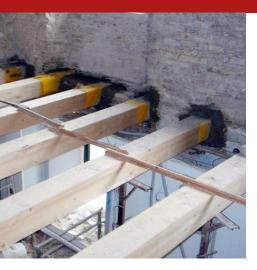
Thixotropic, reinforced fibre, anti-shrink mortar, slightly expansive in plastic phase, high-performance in terms of resistance and waterproofing characteristics, specific for the compensation of cavities and detachments in roughcast underpinning, and for accurate fixing of wooden or steel beams in masonry whatever its nature.
