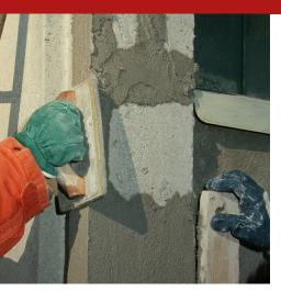
Structural cementitious mortar, two-component, composite, with compensated shrinkage, fiber-reinforced, based on high-strength cements, super-pozzolanic fillers, water-dispersed polymeric resins, migratory corrosion inhibitors, anti-shrinkage additives, plasticizers, stabilizers and anticorrosion agents, selected aggregates, READYMESH microfibers in glass, with a high zirconium content, and multifilament polypropylene.
