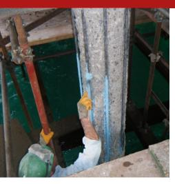
Two-component cement slurry, modified with flexibilising resins and specific anticorrosive agents for the passivating treatment of oxidised reinforcement rods, in the restoration of degraded concrete.
