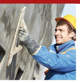
Fine skim, two-component, thixotropic, rheoplastic, composite, "multipurpose", fast solidifying. Perfect for millimetre and cosmetic smoothing of artefacts and works of concrete in structural and/or functional restoration; also suitable for smoothing façades of buildings with partial or total presence of wall plastic coatings.
