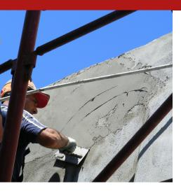
Fine skim, monocomponent, thixotropic, rheoplastic, composite, "multipurpose", fast solidifying. Perfect for millimetre and cosmetic smoothing of artefacts and works of concrete in structural and/or functional restoration.
