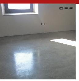
A non-film chemical/mechanical nano-technological hardener with a base of lithium silicates for cortical consolidation, chemical surface hardening and anti-dust treatment of recently-constructed industrial concrete flooring. QL Nano Lithium must be applied on the surface of the floor, immediately after finishing with mechanical bladed trowels. Once the product has been absorbed, it is possible to polish the treated surface using specific polishing machines.
