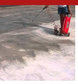
An anti-dust chemical/mechanical revitalising hardener for concrete flooring and screeds, consisting of an aqueous solution of mineral silicates and fluosilicates, activated by specific wetting agents. It is applied in several coats of decreasing dilution in water, with a brush or mechanical "scrubber". Specific anti-dust treatments for industrial flooring or concrete slabs that have lost their original "vitality".
