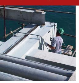
Anti-carbonation, protective, decorative, pigmented paint for painting concrete surfaces, based on acrylic elastomers in emulsion, thermoplastic fluorinated polymers (Teflon), fillerised aggregates, valuable colouring oxides. Perfect for waterproofing, water-repellent painting of artefacts and works in concrete or masonry in harsh environments (marine and mountain environments, chemical industry, steel mills, etc. ).
