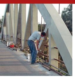
Anti-carbonation, protective, decorative paint, pigmented for whitewashing concrete surfaces; based on acrylic resins in aqueous emulsion, it forms a film that is impermeable to water, with very low permeability to carbon dioxide but high vapour permeability, anchored by specific adherence and diffusion. Perfect for protective coatings of infrastructure projects in concrete.
