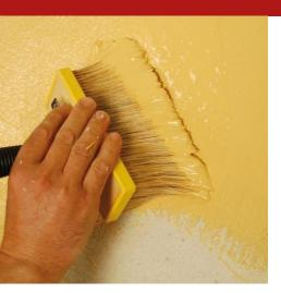
Water-repellent, breathable, pigmented paint based on siloxane resins in water dispersion for painting and renovating civil and industrial buildings, and newly manufactured, for both external and internal facades. Recommended as a breathable, water-repellent protective finish for macroporous dehumidifying plasters (Sanatigh, Sanawarme, Caleosana).
