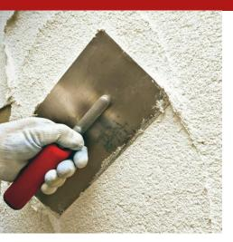
Water-repellent, breathable, pigmented, ready-to-use plaster based on siloxane resins dispersed in water. Ideal for the protective coating resistant to water and bad weather in the renovation interventions, both of external facades and of internal environments, of civil and industrial buildings, and in new constructions.
