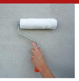
Consolidating, transparent fixative primer based on siloxane resins in aqueous dispersion, specific for the preliminary treatment of plasters before the application of Protech Sil P or Protech Sil P - Therm siloxane paints, or before the application of siloxane plasters Protech Sil I or Protech Sil I - Therm, in the renovation of civil and industrial buildings and in new buildings.
