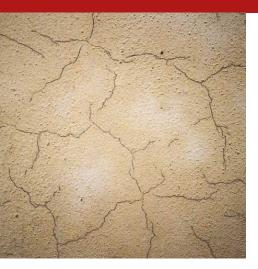
"Anti-crackling" basecoat based on siloxane water-thinnable resins, microfibre nylon, acrylic dispersions, fillers and specific additives, in a special highly water repellent mix ("lotus" effect). The special covering, filling (filler) and vapour permeability capabilities, make it specific for renovating cracklings and small cracks, resulting from plastic and hygrometric shrinkage on existing plaster, before the next painting or coating with putty coat.
