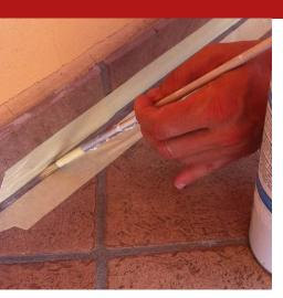
A polyurethane bonding primer for preparing the subsequent filling of the joints with singlecomponent polyurethane sealants in a cartridge (Protech Flex or PROTECH SIGILFLEX MONO) or a two-component product (EG 91) on concrete and masonry surfaces.
