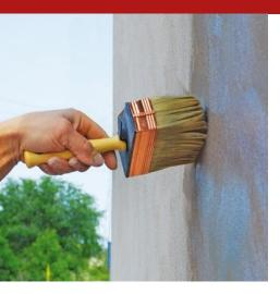
Reinforcing high penetration fixative, non-pellicular, based on ultrafine acrylic polymers with hydrodispersed adhesion promoters. Suitable as a fixative anti-dust primer prior to painting or coating plaster with paints or acrylic putty coats. Used alone, it is a good anti-dust reinforcing cortical treatment of old non-cohesive plaster and jointing.
