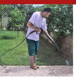
An impregnating water-oil repellent that is colourless, non-film and based on the nanodispersion of silicon compounds. Protects washed gravel floors from the weather, frost and thaw cycles, and aggressive atmospheric conditions. It does not alter the colour of the support nor impact the original appearance or breathability. Also to be used, as a stain prevention during the washing operations of the surface to be deactivated, on the artifacts around the architectural flooring.
