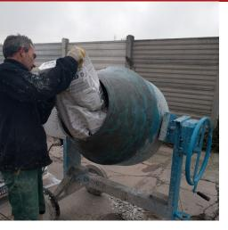
Additive power mix for enhanced performance of the functional characteristics of the concrete used to create architectural floors of landscaping/environmental worth, with a "washed gravel or visible gravel" technique.
