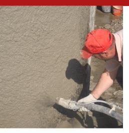
Fiber-reinforced monocomponent cement mortar, based on hydraulic binders, superprogoline fillers, selected fine aggregates and crystallizing reagent agents, which favor the penetration of the compound into the support. Ideal for low-thickness protective coatings (4 to 10 mm), with high counterweight adhesion. The specific formulation makes this product ideal for coatings in aggressive environments in contact with chlorides and sulphates (sewage systems).
