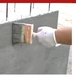
Cement compound for the preparation, with the sole addition of water, of a waterproofing osmotic coating that can create horizontal and vertical barriers, also suitable in conditions of negative hydrostatic thrust vis-à-vis water permeation in the buildings. Typical uses include waterproofing underground rooms, elevator compartments, garages, basements, tanks, etc.
