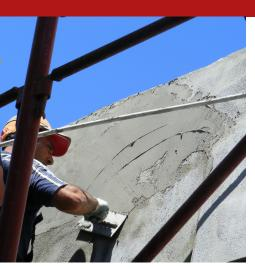
Cement compound for the preparation, with the sole addition of water, of a waterproofing osmotic coating that can create horizontal and vertical barriers, also suitable in conditions of negative hydrostatic thrust vis-à-vis water permeation in the buildings. Typical uses include waterproofing underground rooms, elevator compartments, garages, basements, tanks, etc.
