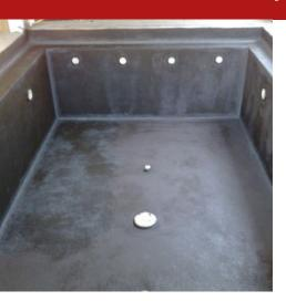
Osmotic cementitious waterproofing from a single-component, fibre-reinforced modified polymer, being super adhesive and deformable, with a plastic-elastic conduct. Ideal for waterproofing beneath tiles and for protecting concrete. It is easily applied by trowel, brush or roller, both on horizontal and vertical surfaces. Offers a 30% higher yield than two-component systems.
