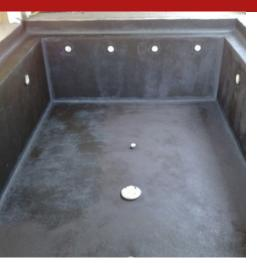
Osmotic cementitious waterproofing from a single-component, fibre-reinforced modified polymer, being super adhesive and deformable, with a plastic-elastic conduct. Ideal for waterproofing beneath tiles and for protecting concrete. It is easily applied by trowel, brush or roller, both on horizontal and vertical surfaces. Offers a 30% higher yield than two-component systems.
