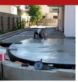
A two-component osmotic cementitious waterproofing agent in water dispersion, being a modified polymer that is highly flexible and deformable, with a plastic-elastic conduct. Application by trowel, brush or roller. Ideal for waterproofing terraces, balconies and swimming pools, prior to laying the tiled or brick coating. Suitable for contact with drinking water.
