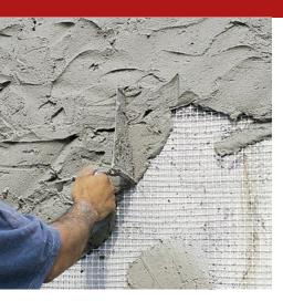
Plaster, premixed, fibre-reinforced, based on hydraulic binders with a low content of soluble salts, for reinforced plastering, bedding of bricks, plastering, repair and covering of internal and external walls and masonry, repair of concrete elements.
